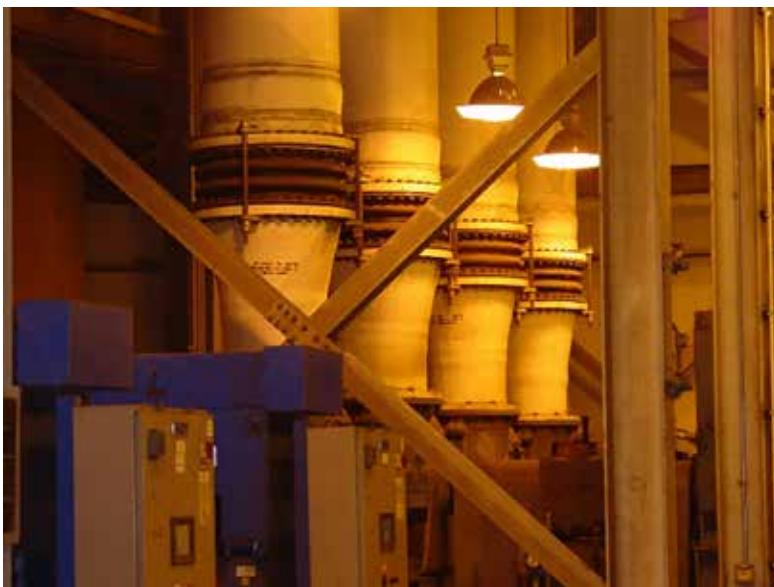
IMAGE 2: Expansion joints installed in nonmetallic piping system
